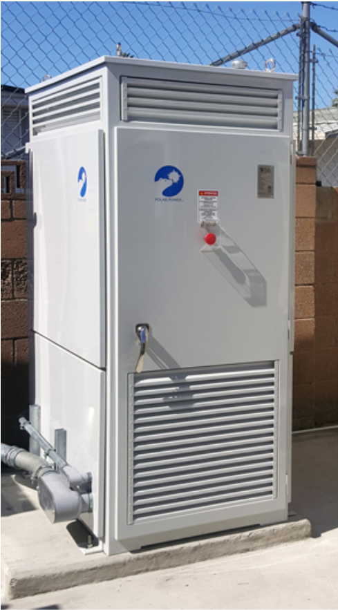
Polar 15 kW diesel backup DC power system
