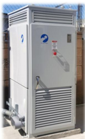
Back-Up DC Generator Solar Hybrid
